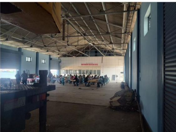
Figure 10: Inside view of Godown
