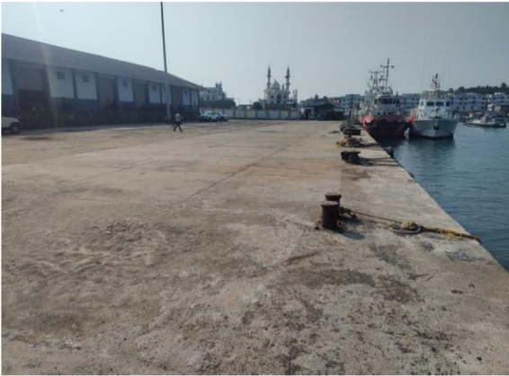
Figure 3: Seaward Wharf with Tugboat tied
