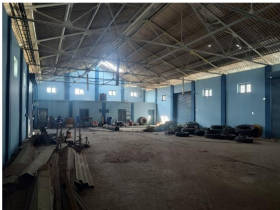
Figure 9: Inside view of Godown
