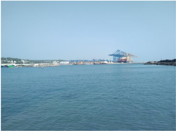
Figure 4: View of Vizhinjam International Sea Port from Wharft
